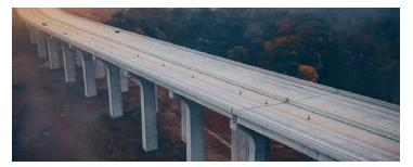
**The Prestressed Concrete Stringer Bridge** Became one of the most dominant bridges since its creation. The bridge consists of a series of reinforced concrete beam parallel to the deck that support the structure. [1]
