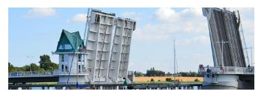
The Bascule bridge or (Drawbridge) rotate in a vertical plane. They main purpose is to be able to rise and lower allowing ship to past under the river. [1]
