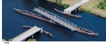
The Swing Span Bridge rotates in a horizontal plane around a vertical axis in the water. This allows the movement of ship and other small boats. [1]
