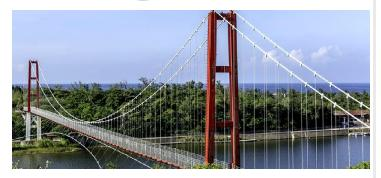
The Suspension footbridge consists of cable which help support the structure. These Cable are usually under high tension. [1]
